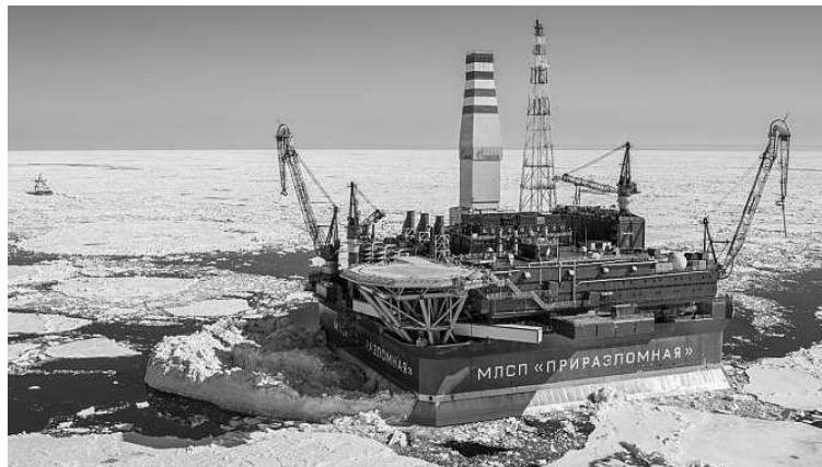
Fig. 6. Gravity base offshore oil rig in ice pack
